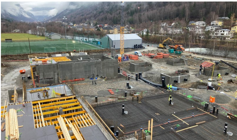
Overview of facility
