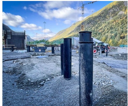
Pipes under ground ongoing
